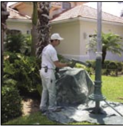
Electrostatic application of finish coat to base of light pole
