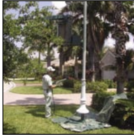
Glass light fixture is masked off and white primer is applied
